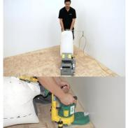
Sand the floor with a Belt Sander and a sanding belt P40. Depending on the type and pattern of the floor sand at a light angle or diagonal.
