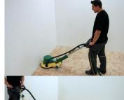
Use a single disc machine with a LOBATOOL Perforated Pad P 100 alternatively a sanding net P100 and sand along the walls as close as possible to equalize the transition from edge sander to belt sander.
