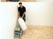
Perform the final cut with the belt sander and sanding belts P 120 into the direction of the wood. Drive as close as possible to the walls.
